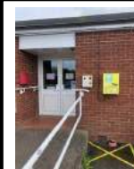
Parish Hall HR1 3LJ
