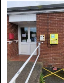
Parish Hall HR1 3LJ
